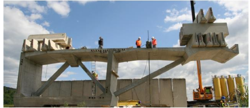
Composite bridge segment load test - Extradosed Viaduct Pov. Bystrica
