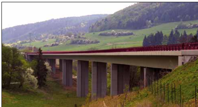
Obr. 1 Most D 214 Fričovce
